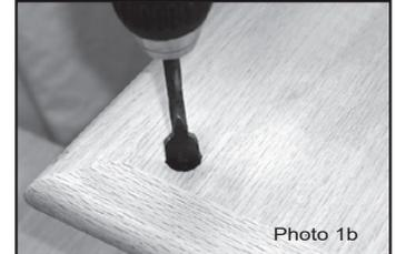
2. Refer to the Key above and drill a hole 3/4" deep on each tread at each marked baluster location. (Photo 1b)
