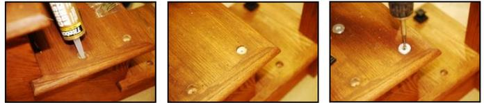
(For new stairway construction, place the threaded disc over the baluster centerpoint and install into the tread using the 1 1/2" Attachment Screw)
